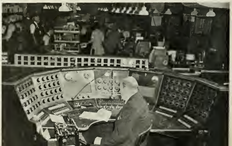
LEFT: AT OPERATING POSITIONS SUCH AS THESE, RCA MESSAGE TRAFFIC FLOWS TO AND FROM VIRTUALLY EVERY IMPORTANT SECTION OF THE WORLD. BELOW: TECHNICAL CONTROL OVER MORE THAN FIFTY INTERNATIONAL RADIO CIRCUITS IS MAINTAINED AT THIS DESK IN RCAC'S CENTRAL OFFICE IN NEW YORK.
