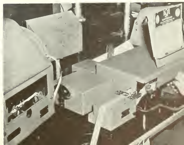
BELOW: HIGH-SPEED MULTIPLEX RADIO-TELEGRAPH PRINTERS TRANSMIT MESSAGES ACROSS THE SEAS AT THE RATE OF HUNDREDS OF WORDS A MINUTE.
